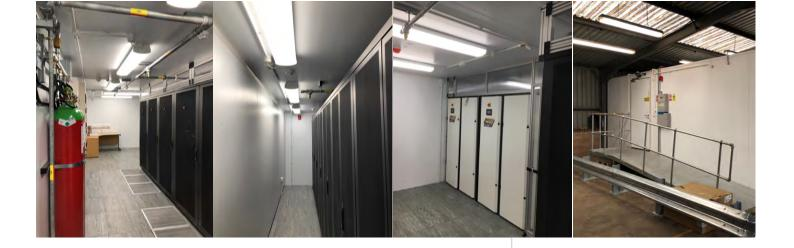
To address the proximity of the data centre to vehicles and fuel storage it was imperative that the building was suitability protected. Workspace Technology selected ModuSec the UK's industry leading fire rated pre-engineered composite panel system to optimise protection of their IT compute equipment from fire, heat, water, smoke and attack. The building was also protected by a secondary vehicle barrier around its perimeter.
