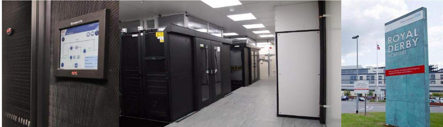
The initial stage was the construction of the 'white space' to house the critical IT infrastructure. This was formed using a modular composite panel system, that provides 60 minutes of fire protection, along with the installation of raised access flooring throughout using heavy grade computer room tiles.
