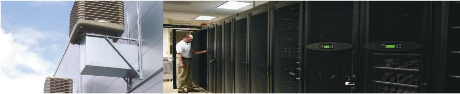
into the data centre cold aisles. Hot air is drawn out of the hot aisles by a series of fans into the upper level 'hot chamber' where it either exits the building or is recirculated dependent on external ambient air temperature conditions.
